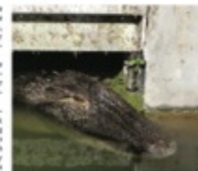
This 7-foot-3-inch alligator found its way into the contact chamber of the city's waste water treatment system last week.
