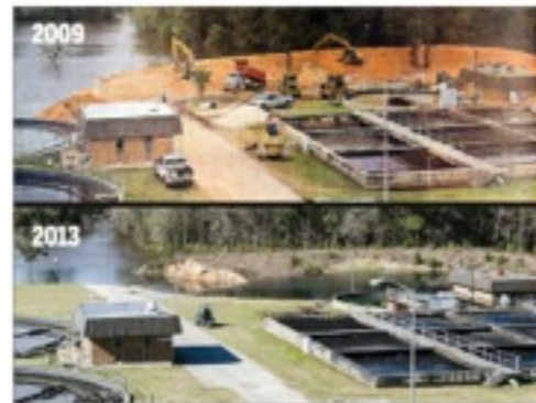
A 2009 photograph (top) shows the construction of a berm near the 10th station (the right building) at the waste water treatment facility. The bottom photo, taken Thursday, shows a significant portion of the berm no longer visible, allowing floodwaters to reach the 10th station.
